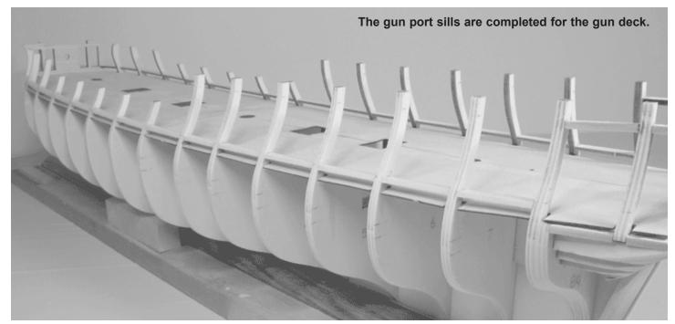
the hull using the reference marks you made. Mark each side of the sill with pencil and cut it to length. Don't make the sills too tight or you will force the bulkheads out of alignment. They should be a good close (snug fit). Line up the top of the sill pieces with your reference marks. When all of the sills have been glued into position, you can fair them until they are flush with the bulkheads. See the photo provided.
