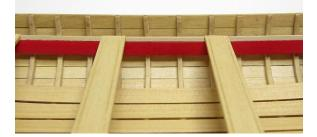
basswood strips between the thwarts (just above the riser). See the photo provided that shows these strips glued in position. They will need to be pre-bent to accommodate the curved bow.
